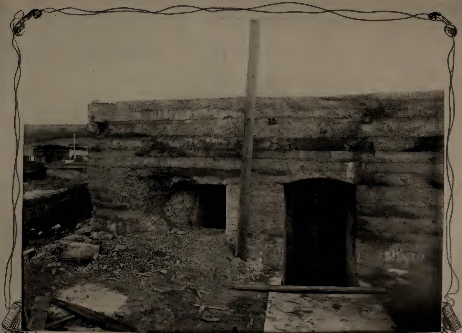
Direct hit on pill box at Vilosnes.
